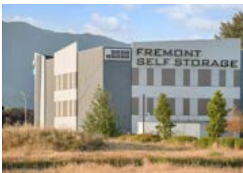
PORT COQUITLAM, BC
